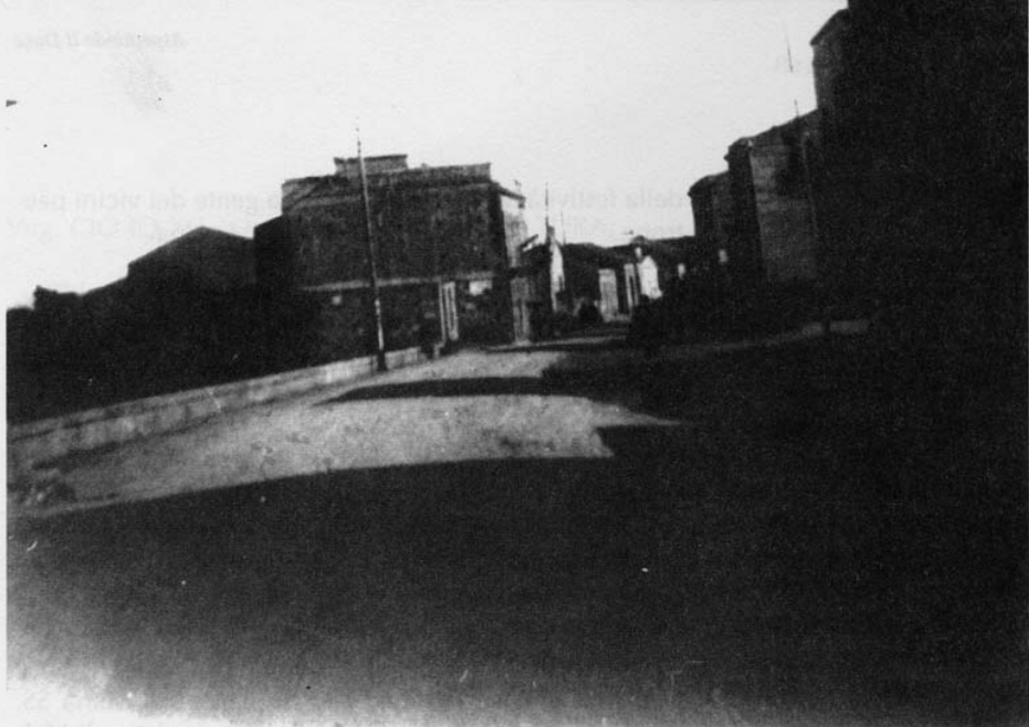
Left is the entrance to the... The photograph is a... The photograph is a...
